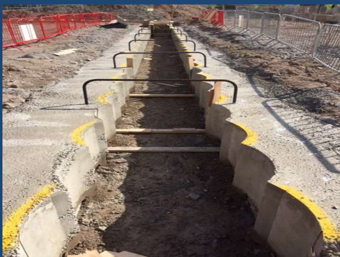
Installing Secant Guide Wall
