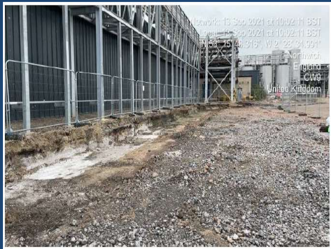
Excavation for Retaining Wall
